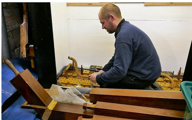
Simon Tipping working inside the Swell box at Kirk Langley, reconnecting the wind supply to off-chest pipes.
