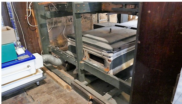
The reservoir at Shirley with trunking removed. The colourful unit to the left of the photo is the humidifier, the purpose of which is to stop the leather and wood drying and cracking in a well-heated building.
