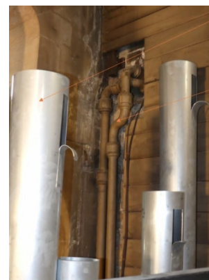
Unlagged heating pipes detrimentally close to reed pipes!
